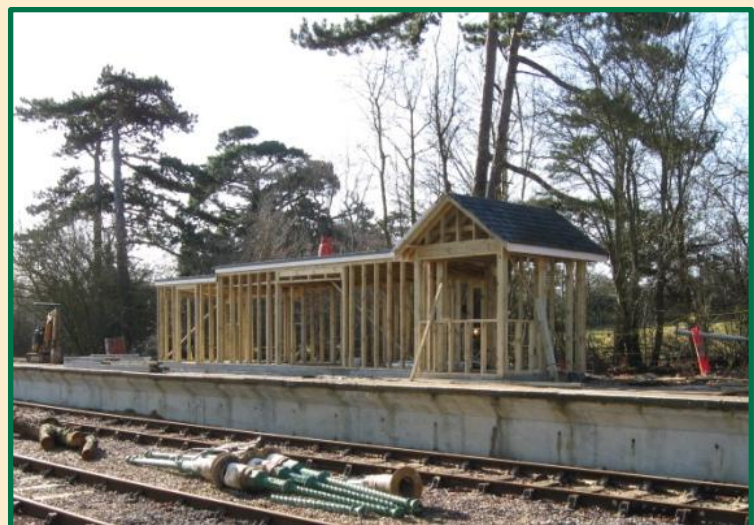
Progress as at March 2012
